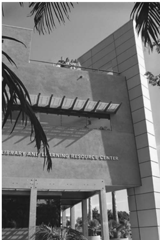
View from the top of the Library and Learning Resource Center.
