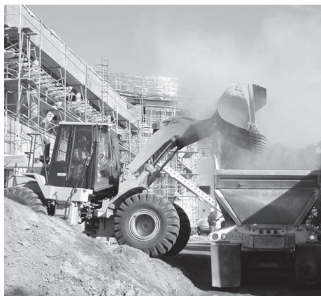
Backhoe raises dust during construction of LRC Nov. 2003.
