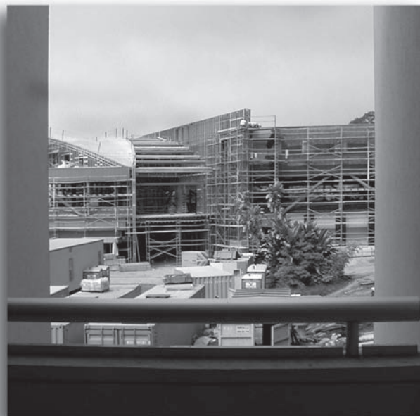
Library and Learning Resources Center from science building
