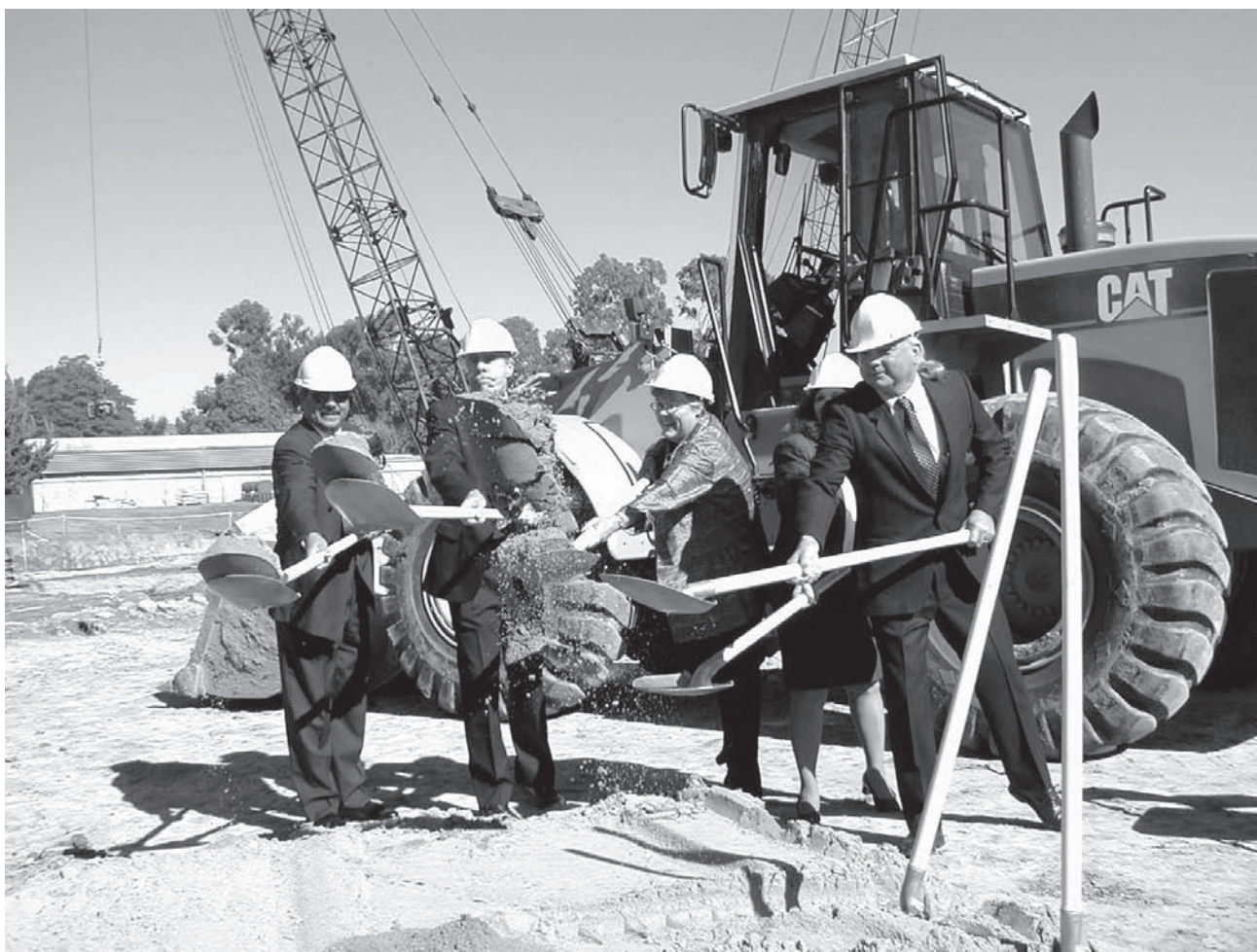
Groundbreaking for the new LRC, Sept. 2002, left to right: former President Larry Calderón; former Interim Chancellor Jim Walker; Dean Diane Moore; LRC Supervisor Sandy Hajas; Professor Larry Manson
