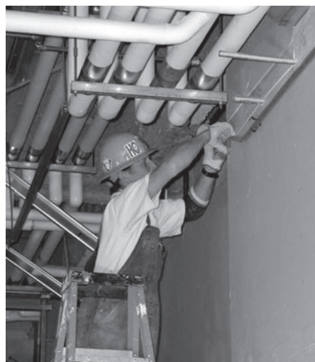
VC Alum works on the LRC electrical system
