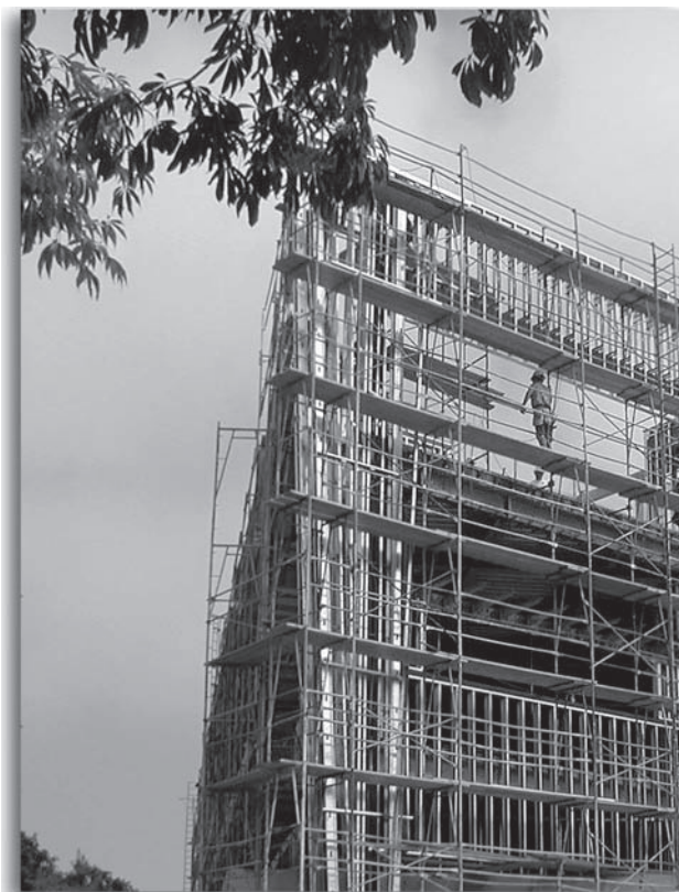
Constructing the LRC building, Sept. 2003.
